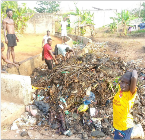
Blocked culvert
